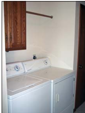
View of Laundry Area
