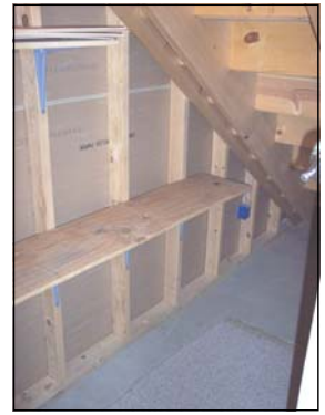
View of Storage Under Stairway
