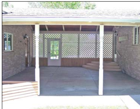
View of Roof-Covered Patio
