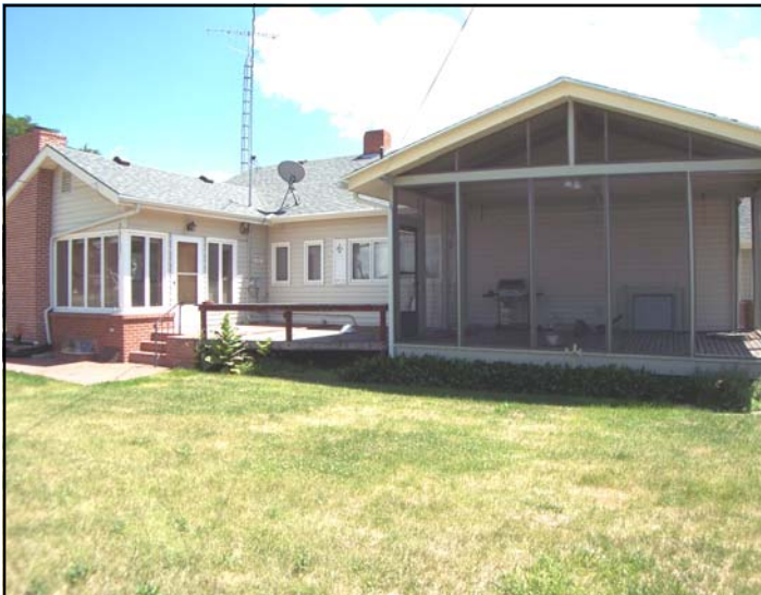
Back View of House
