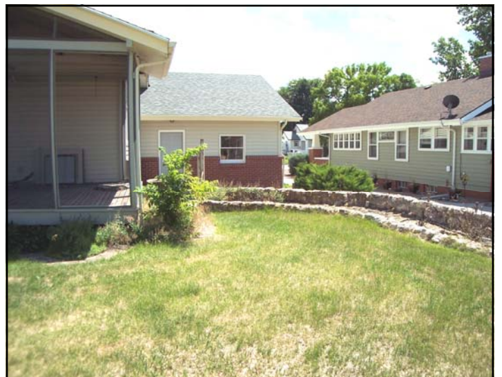
View of South Side of House
